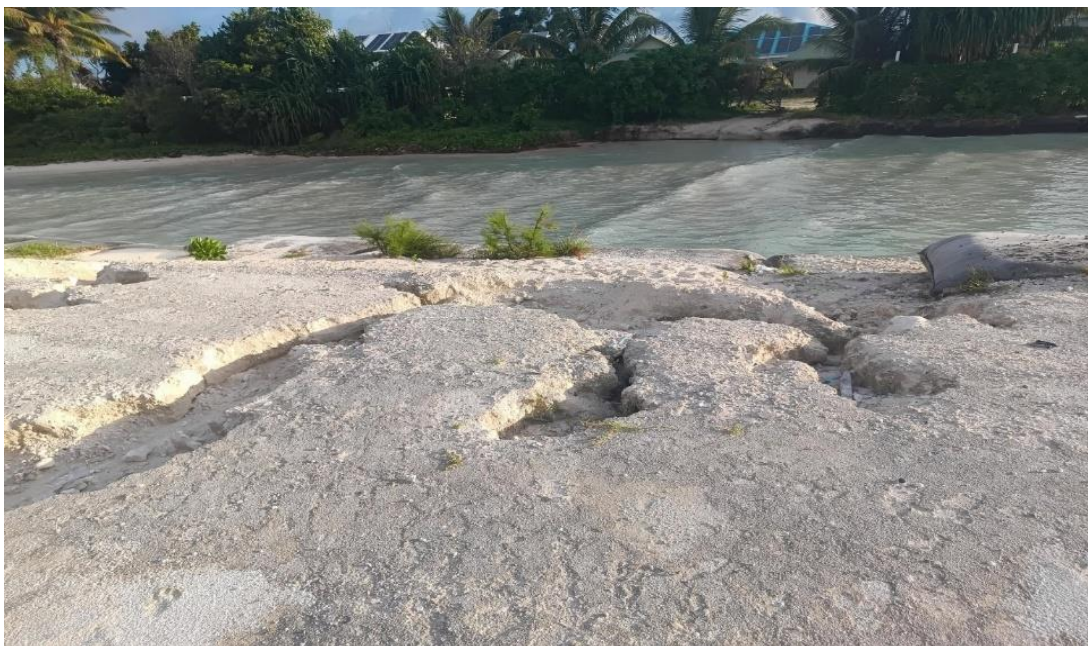
Figure 11. Rills caused by heavy rain (auditors)
