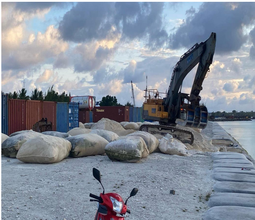
Figure 9. Geosynthetic sand containers being replaced with new ones by the HALL company.
