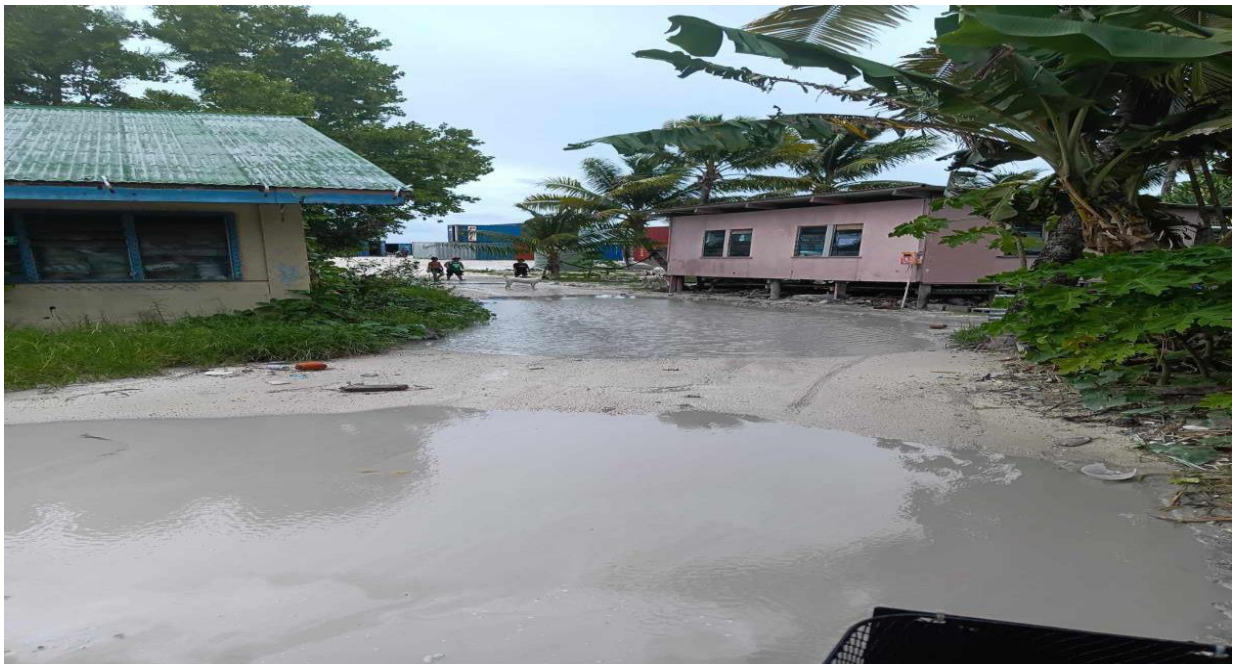
Figure 12. Flooding outside homes adjacent to the main access road to the reclaimed land, caused by potholes filling with rain water during heavy rain (auditors)
